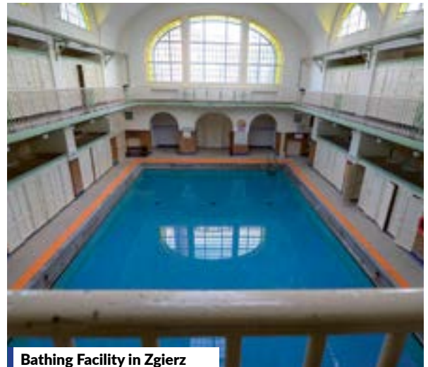
Bathing Facility in Zgierz
